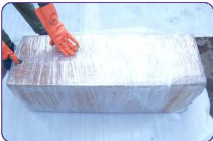
Unbox the carton of backflush assembly carefully with the help of knife/cutter
